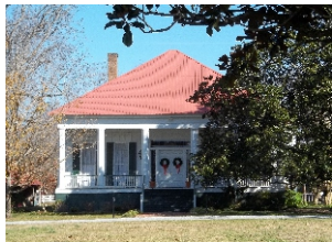
2. River Bluff House
